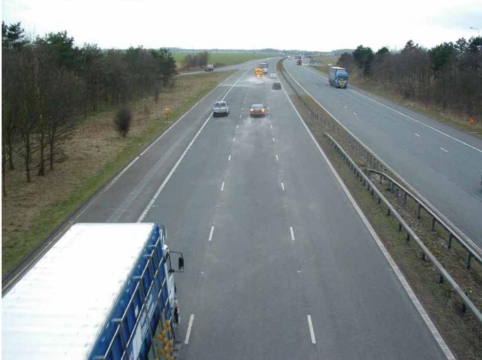
**Figure 3.11.4 - Displacement of de-icer by turbulence from vehicle draughts immediately after spreading**
